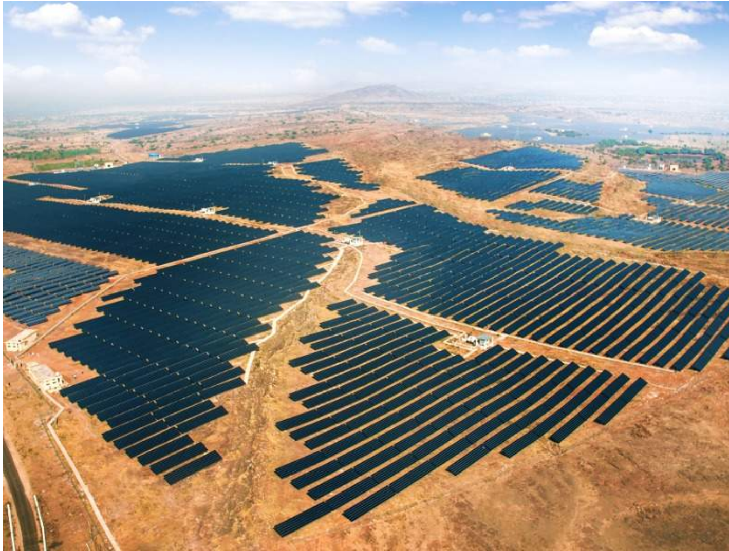
Biggest solar farm in the world: Bhadla Solar Park, Rajasthan, India: total installed capacity of 2,245 MW, spread over a total area of 5,700 ha
