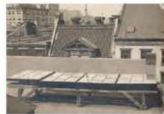
The first solar array installed by Charles Fritts in 1884 in New York City. Fritts built the first solar power in 1884, reporting 940 in the current solar "conversion" and that kind of solar devices that can only be replaced by
